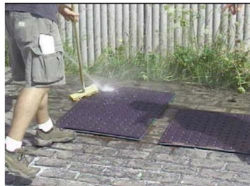
4) Day two – If desired, take a scrapper and knock off any tips from the domes that are extreme. Then wash residue left from Liquid Release off surface using a mild detergent and water.
