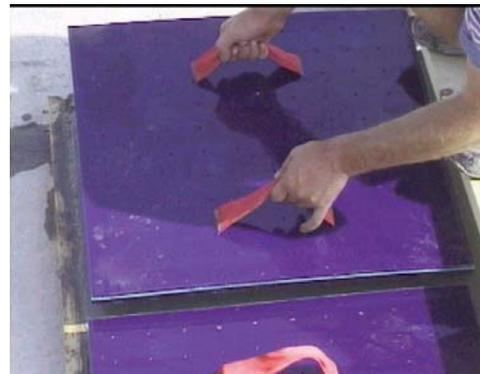
3) Tamp the stamping tool and make sure to cover every row of the domes in order to achieve the proper design and appropriate number of domes. Then lift stamps straight up, being careful not to drag and wash off any concrete that may have stuck to the stamps.
