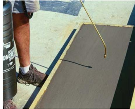
2) Use plank to bridge surface to be imprinted and place stamps on surface from directly over top. Do not drag or pick up the stamps after placing them on concrete.
