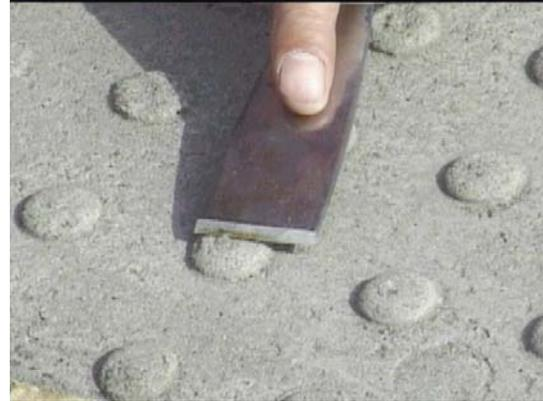
5) Apply 2 Coats of ADA Colour-Seal to desired surface when dry to give the light on dark contrast and you have your completed project.
